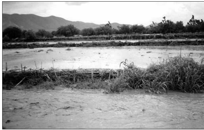
Figure 3. Dikes of wood stakes and stone built perpendicularly to the slope.
