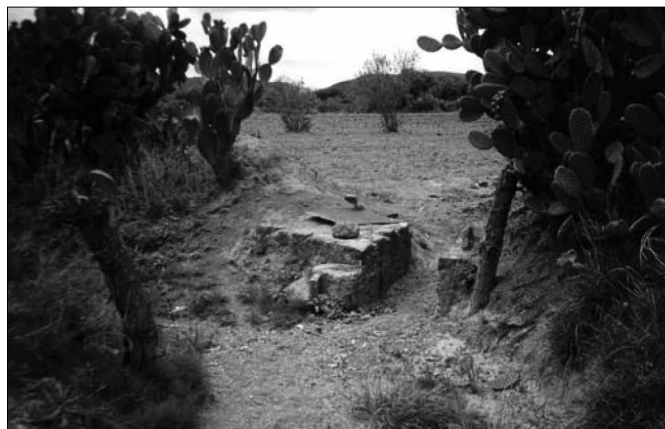
Figure 5. Dispersion of water through smaller dikes built of soil and stone.
