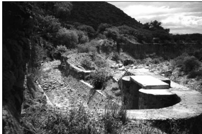
Figure 4. Diversion dikes constructed along a stream.
