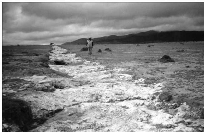
Figure 2. Intercepting and channeling the runoff from the surrounding hill side towards the fields in the bottomlands.
